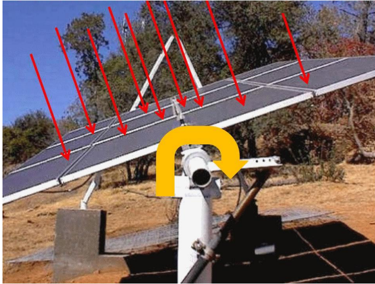
Picture 1. A variable angled array rotating perpendicular to the arriving energy (2)
